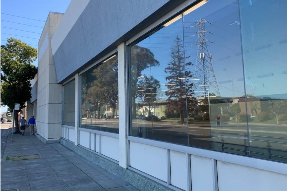
Figure 5. Detail of east elevation aluminum frame windows and stucco cornice, view looking southeast.
